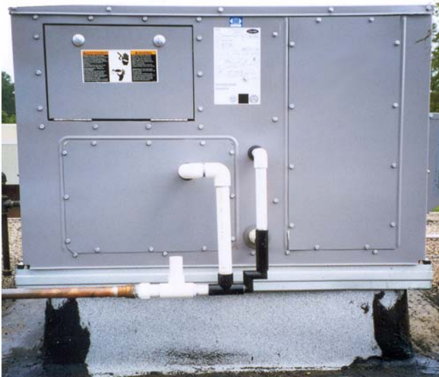
The Fluidic Flow Control Device replaces the condensate P-trap. It is self cleaning (no flow blockage) and self regulating. With this device, facilities managers can achieve dry and clean HVAC systems.
